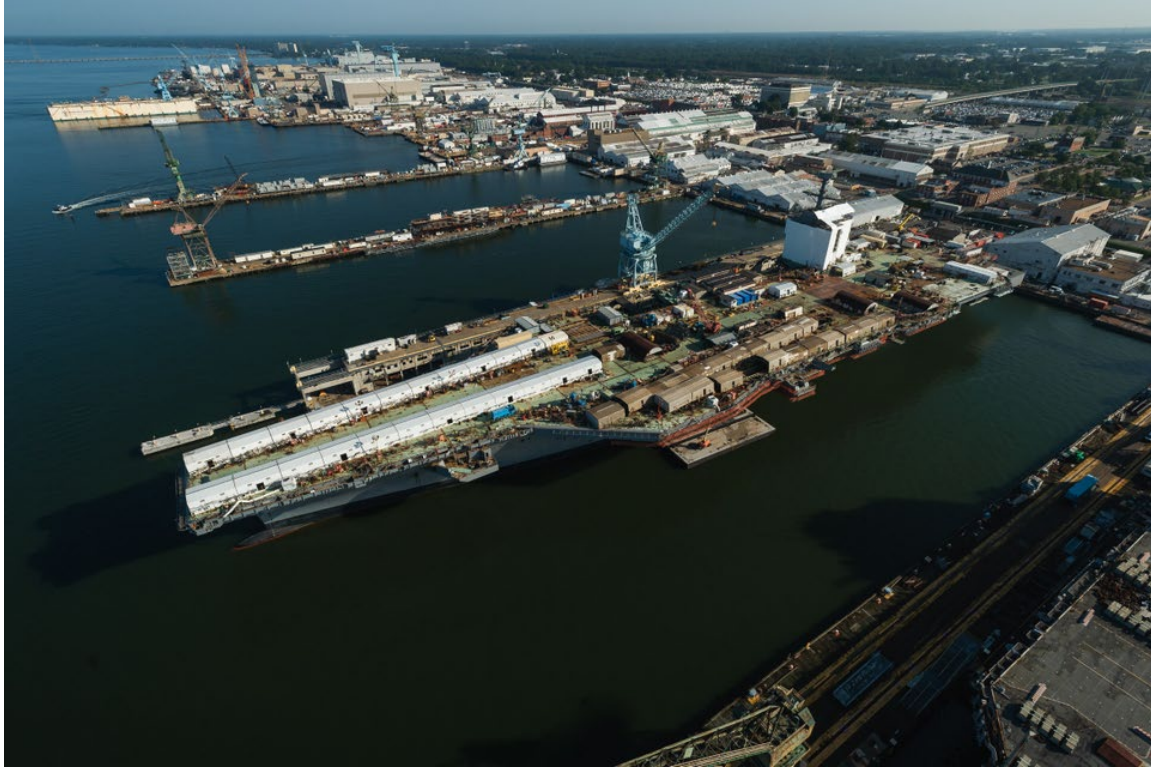
Figure 18. USS John F. Kennedy (CVN 79) sits at Newport News Shipbuilding on 02 November 2020, approximately 76 percent complete and progressing through final outfitting and testing. Source: Hildreth (2020).
