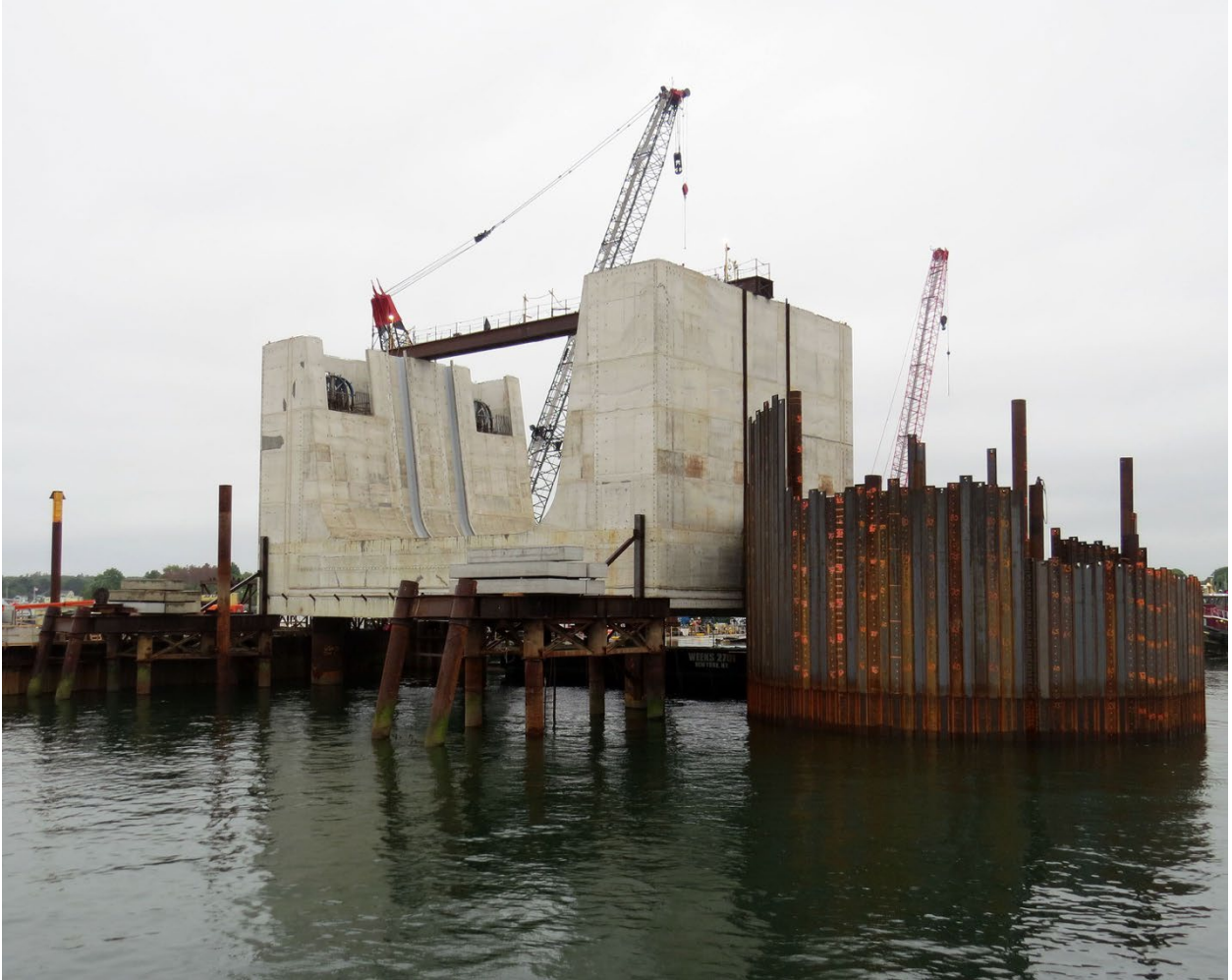
Figure 4. A precast entrance basin is positioned prior to lowered at the Portsmouth Naval Shipyard. The new entrance basin will support the Navy's future fleet of submarines. Source: Eckstein (2022).
